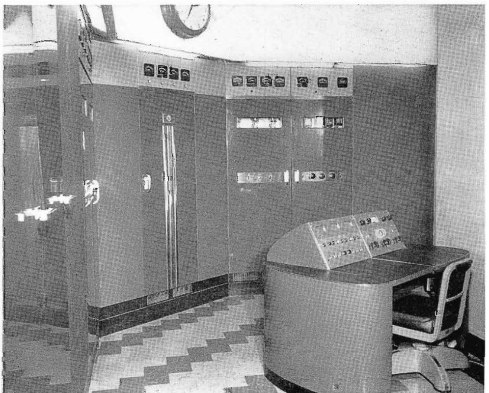
FIG. 12. The model of neat, flush construction is shown in this photo of WMAR-FM transmitter room. Station uses 10 kw RCA FM transmitter which feeds a two-section Pylon Antenna.
