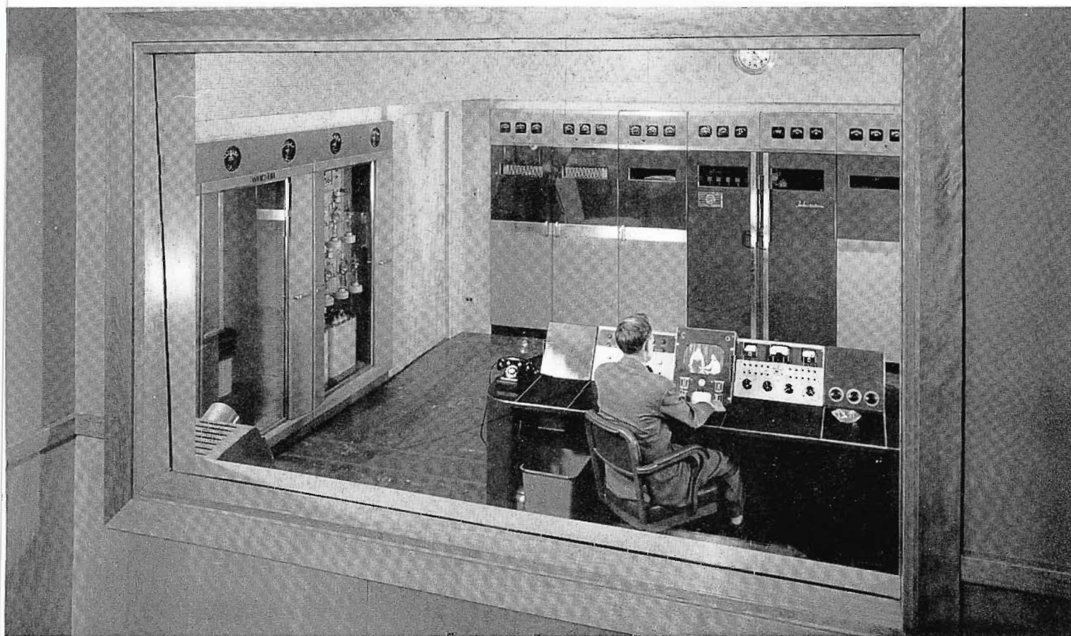
FIG. 6. View from lobby into transmitter control room. FM transmitter is at left, RCA TV transmitter in center.
