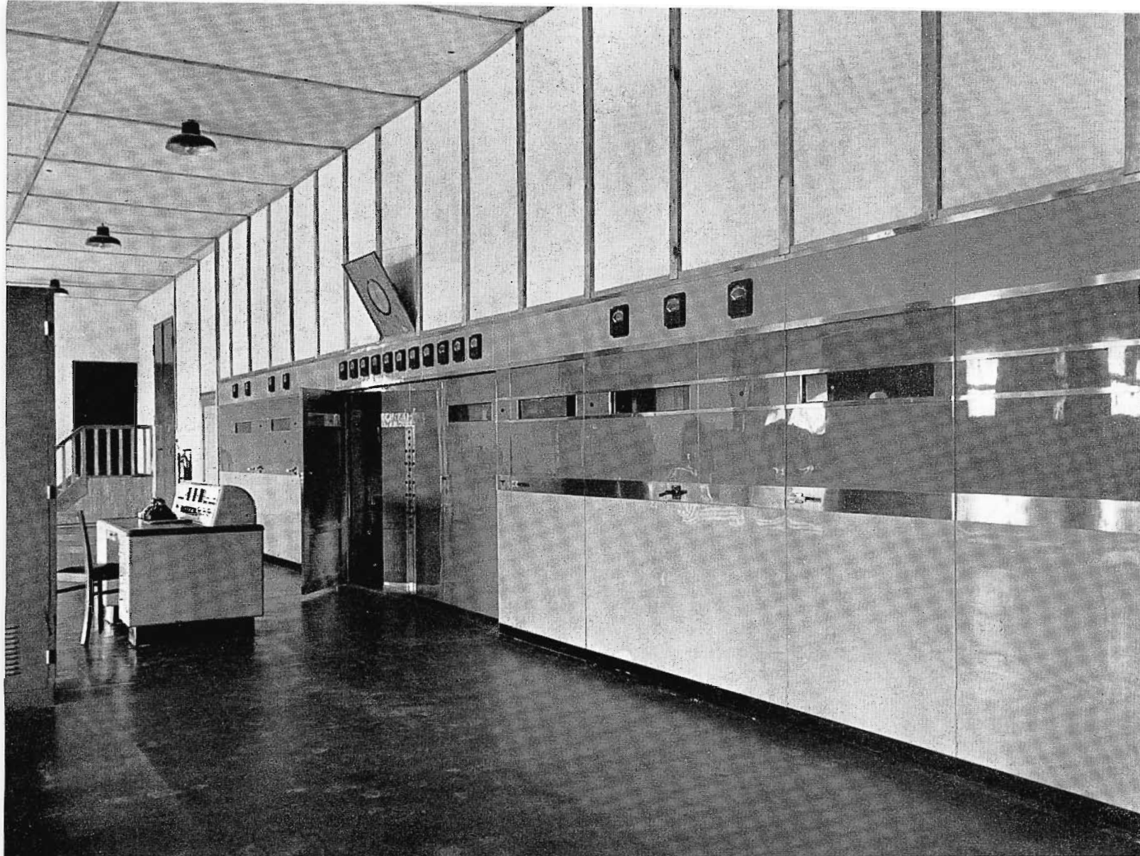
FIG. 1. Front panel of the "Voice of America" transmitter as seen from right side of room.
