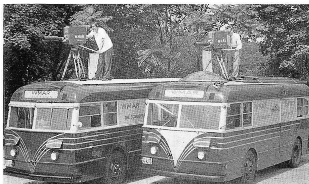
FIG. 15. These custom mobile units carry the necessary field gear for WMAR's heavy schedule of remote telecasts.
