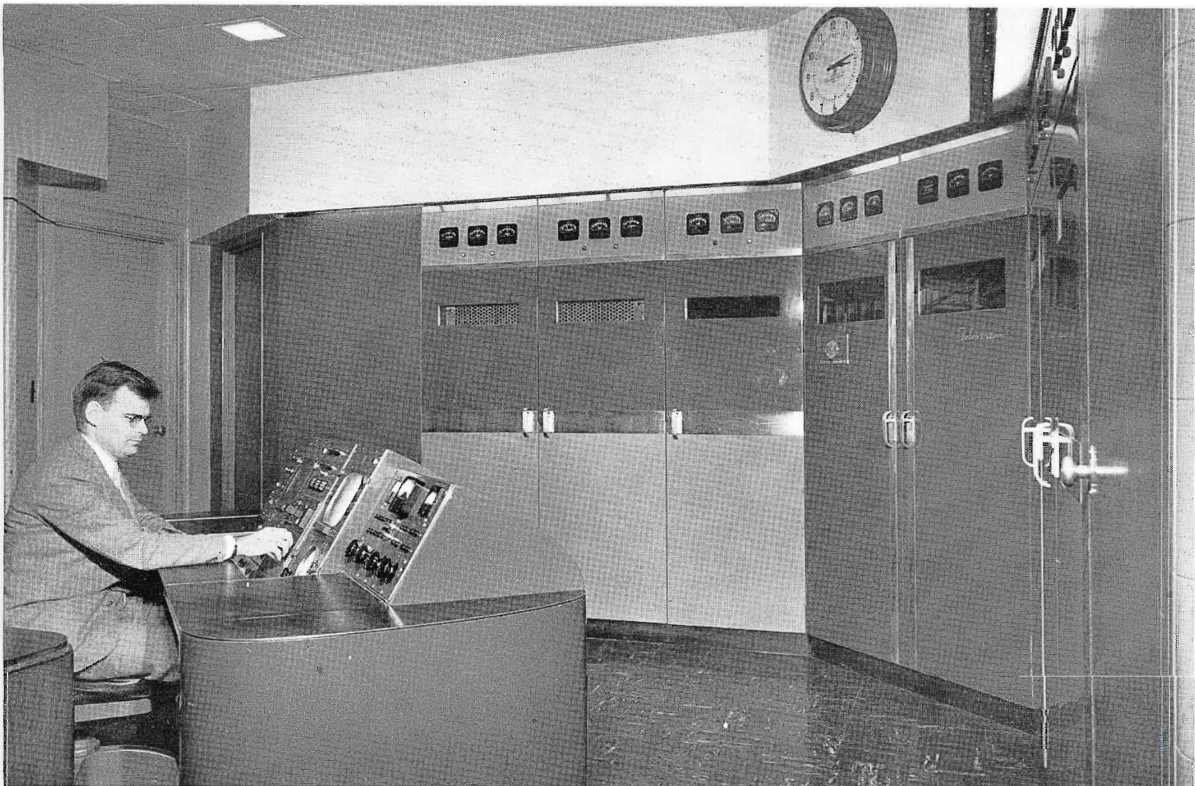
FIG. 10. C. B. Lau, Television Transmitter Supervisor, checks picture quality on TV transmitter control console. Note "U" arrangement of RCA TT-5A TV Transmitter.
