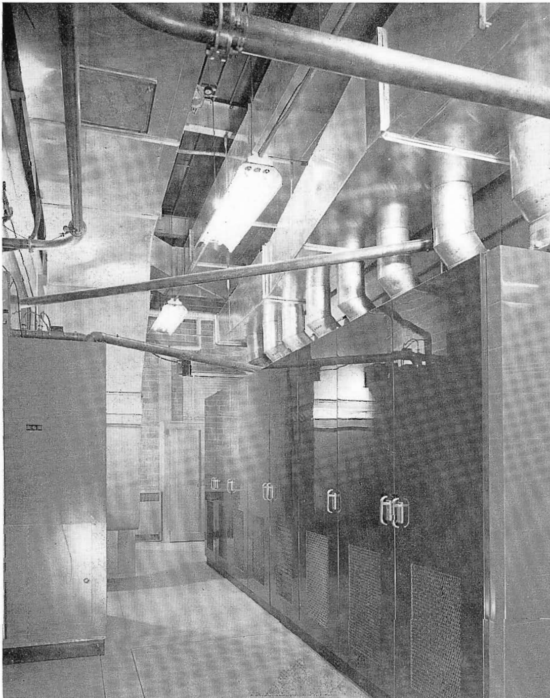
FIG. 15 (left). Scene behind the TV transmitter at WHIO-TV. Each transmitter cabinet is separately vented to the main exhaust duct. The side band filter can be seen on the extreme left, while the FM transmission line is enclosed in the conduit in the foreground above. A special 7,850 cfm. ventilating unit in the left background presently serves the studio and other areas which have been designed for future air-conditioning.
