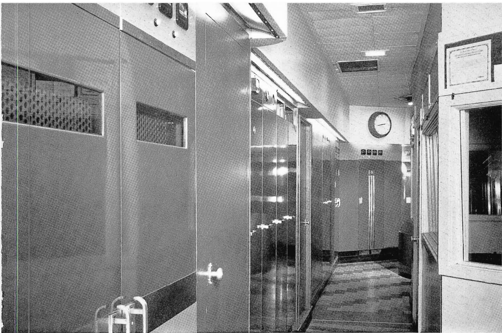
FIG. 11. Line-up of equipment around skyscraper tower presents this impressive array when one looks down corridor from TT-5A to the RCA 10 kw FM transmitter at opposite end.
